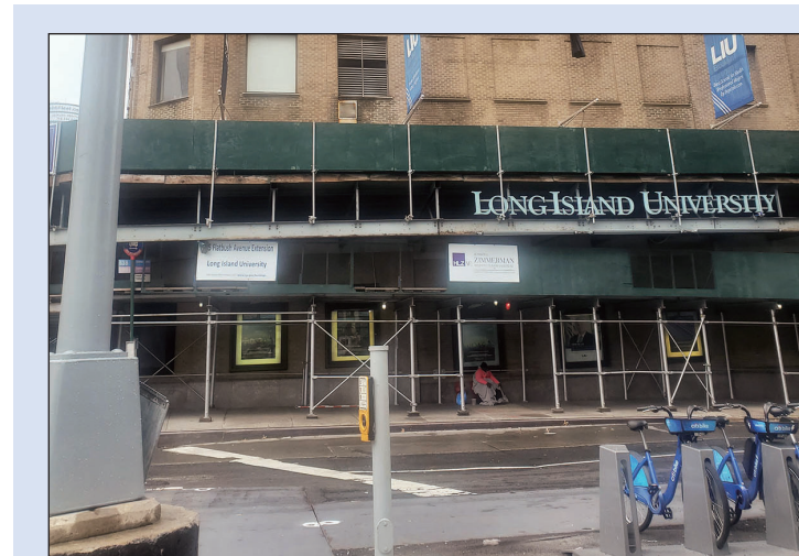
The scaffolding above the Metcalfe entrance to LIU provides shelter for the ever-growing homeless community (Photo: Mymuna Islam)
